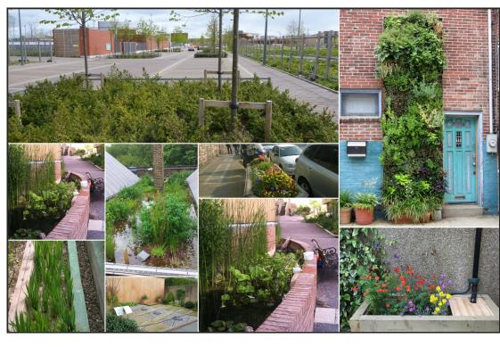
Raingardens are vegetated features which hold rain or surface water, slowly releasing it, helping to reduce the likelihood or severity of flooding.
