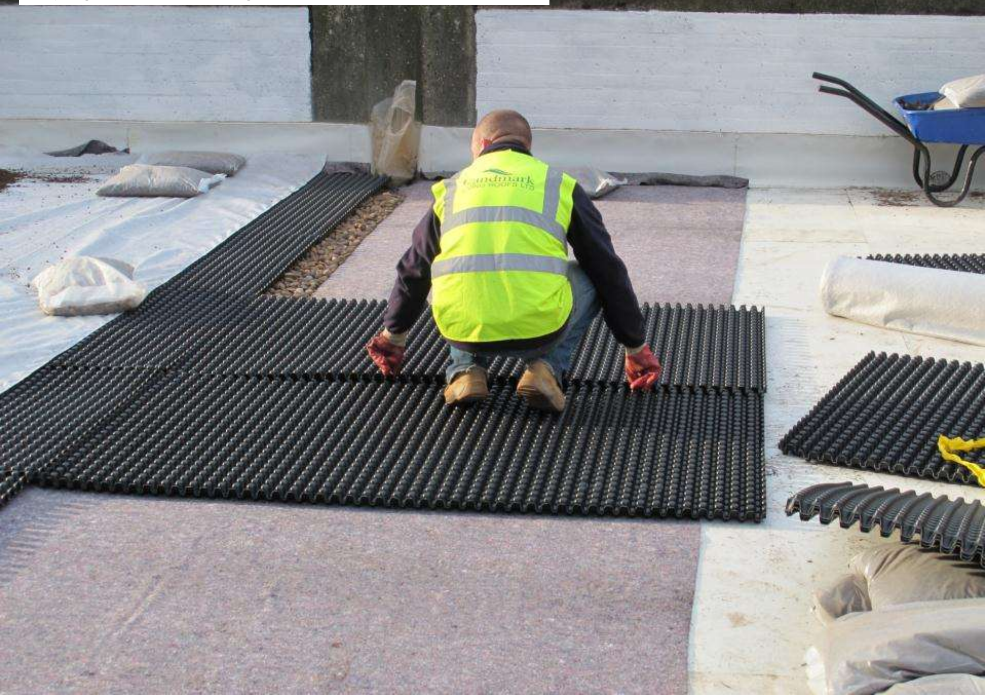
Laying down of drainage board on top of root barrier
